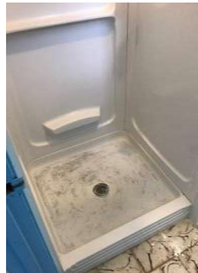
Final Cement Floor
