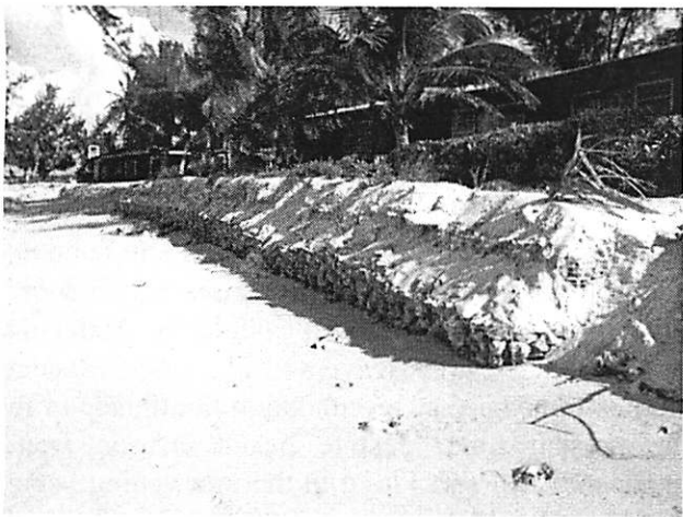
Figure 6. Rebuilt sand dune with young vegetation showing resistance to summer wave action.
