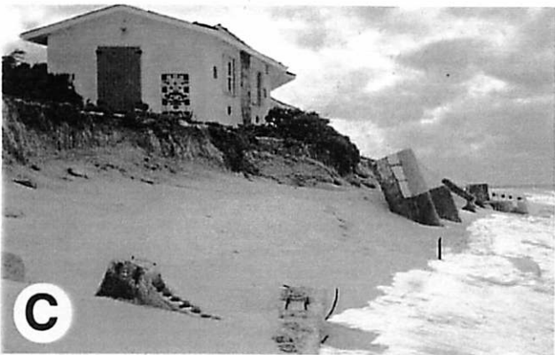
Figure 6. Storm erosion effects in Area 4 – Grotto Bay to Sandy Point: A) Severe beach erosion and scarping immediately south of the section of rocky coast at the south end of Grotto Beach. Note exposed beachrock and the steep scarp cut by wave erosion. B) A continuous scarp was cut into the dunes along the northwestward-facing beach between Grotto Bay and Sandy Point. C) The Savio house viewed from the north; note the remnants of the seawall destroyed by Hurricane Floyd and the vulnerable position of the building's foundation. On this day in January 2000, a weak northwest storm had generated waves that were washing to the base of the scarp. D) Savio house as viewed from the south on a fair-weather day in January 2000.
